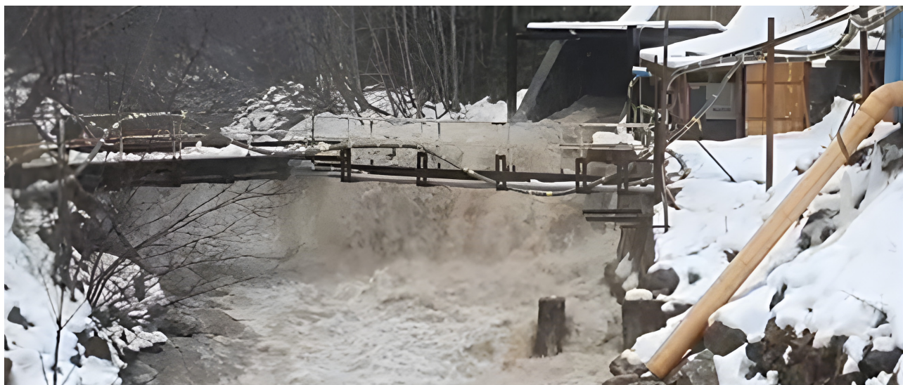
13 End of the 2023 season before dismantling of outdoor installations
