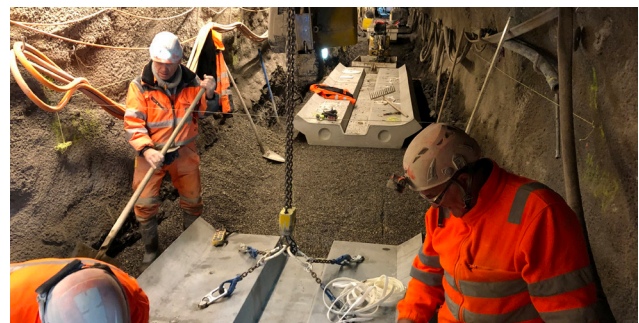
12 Installation of invert segments using the monorail
