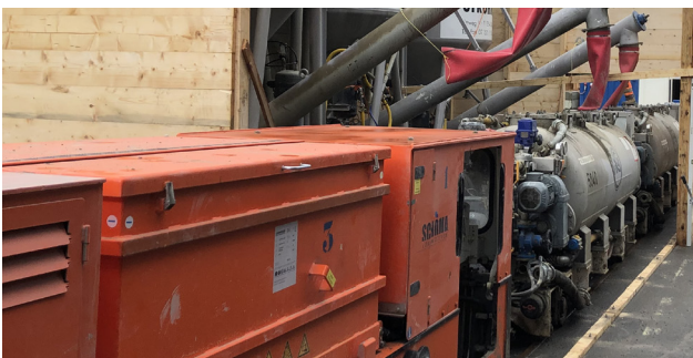
11 Loading of the shotcrete train
