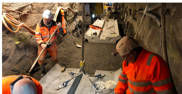
12 Installation of invert segments using the monorail
