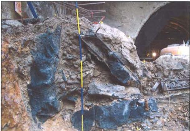
placed in the bench left wall, guided by a dipping discontinuity inwards the tunnel wall. It is important to mention that all calculations indicated that the rockmass behind the bench side walls was overload due to the structural tunnel model and construction procedures and sequence.
