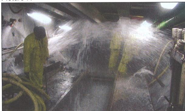
Ground water pressures could reach 27 bar under the maximum ground cover.
