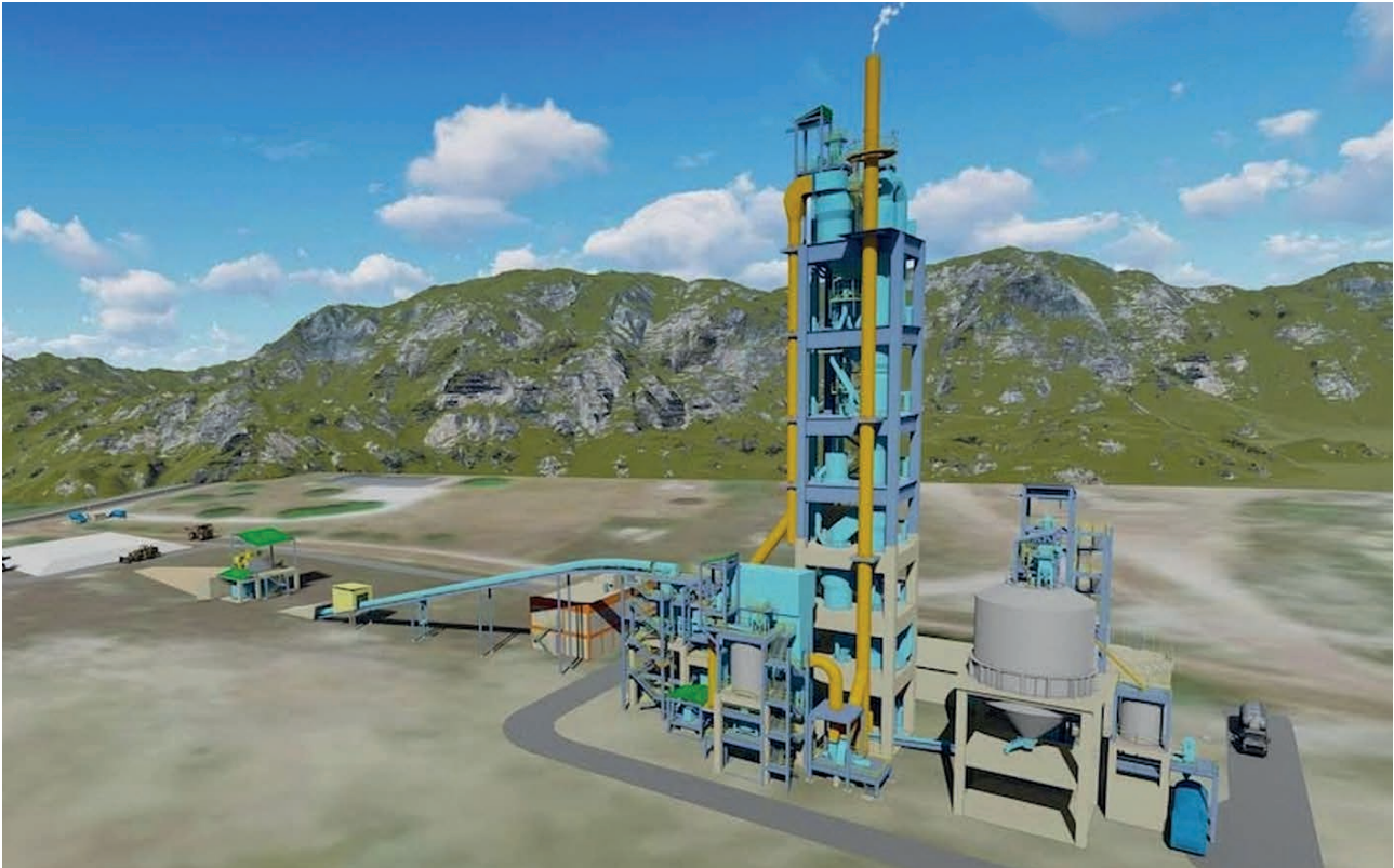
6 3D isometric view of a flash calcination plant for clays
